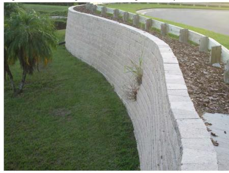
Vegetation on wall along south side Winding Stream Way at round-about
