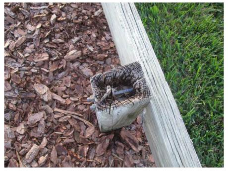
Deteriorated posts in guardrail at round-about
