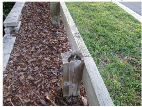
Deteriorated posts in guardrail at round-about
