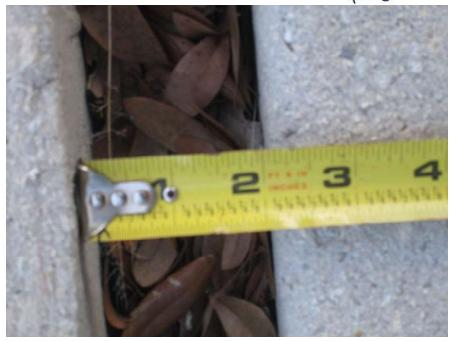
2" Gap between curb and sidewalk at west side of round-about
