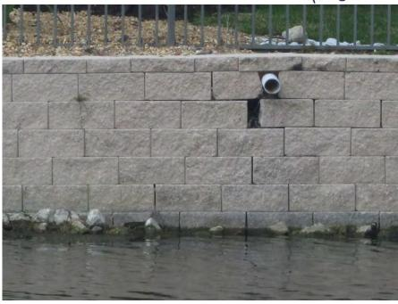
Drain pipe between lots 9 & 10 and damaged blocks with gaps
