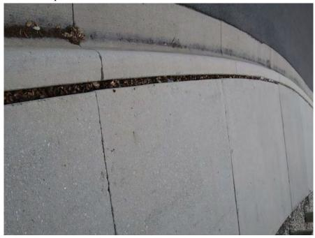
1-1/2" Gap between curb and sidewalk at east side of round-about
